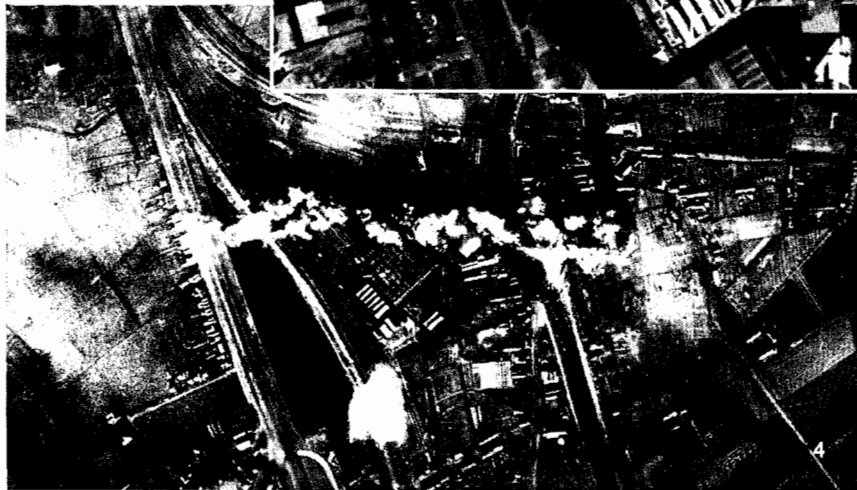
THE STORY OF A BOMB RAID: 1. 4,000-lb. block-busters awaiting disposal over Germany. 2. The men who carry them to the German cities. 3 and 4. Two examples of extensive bomb damage.
