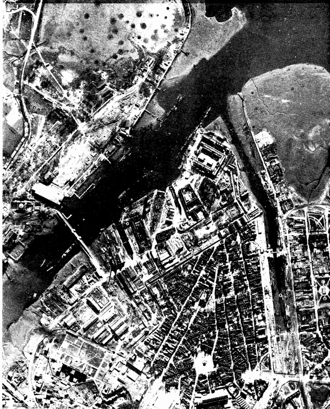
Lorient, France, showing heavy bomb damage.
