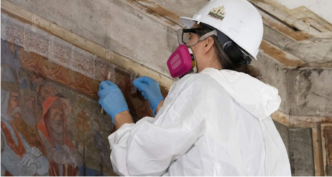
Restoration work at Centre Block
