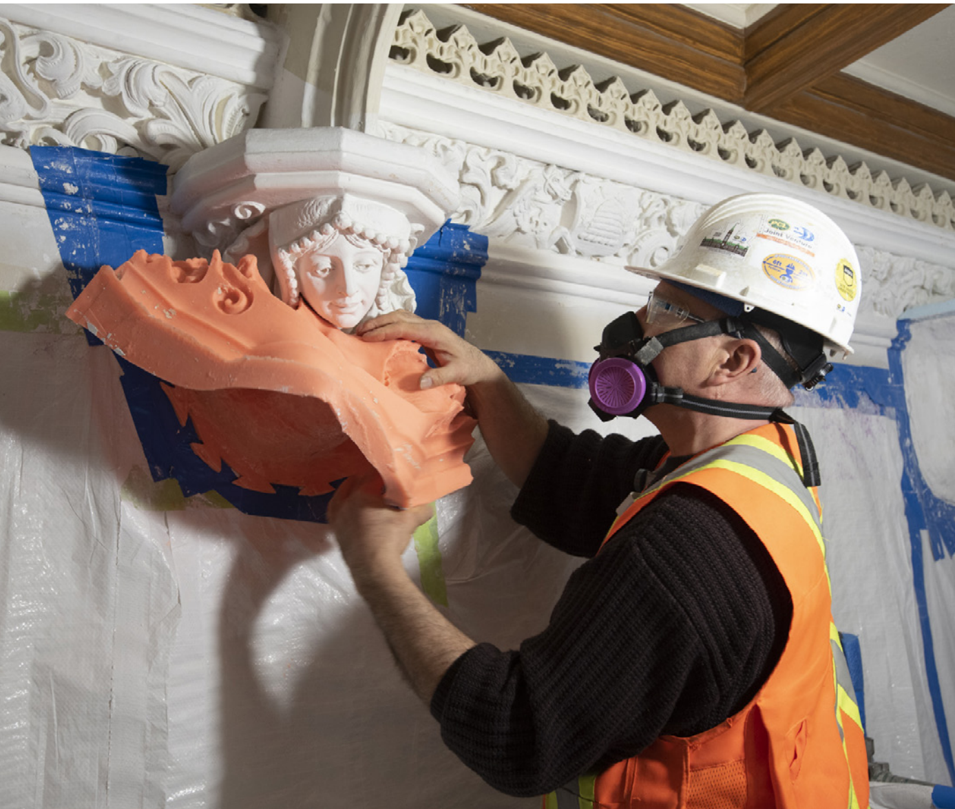
Parliamentary Precinct renovations
