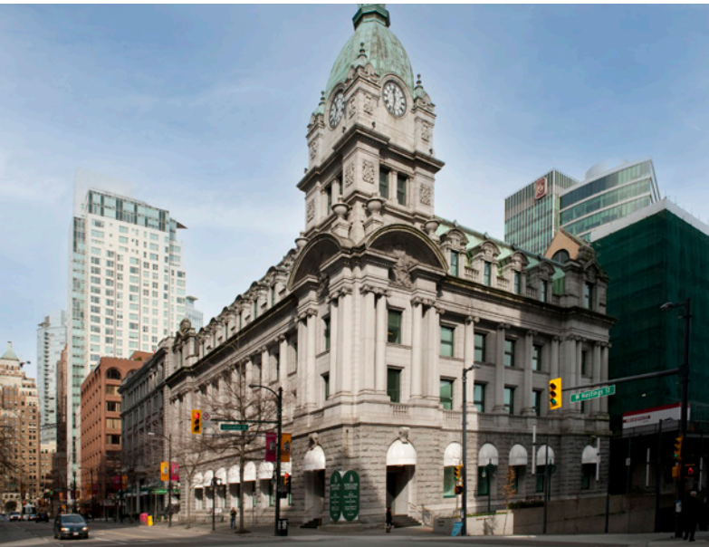
Within the Pacific Region, PSPC will rehabilitate and redevelop the Sinclair Centre in downtown Vancouver
