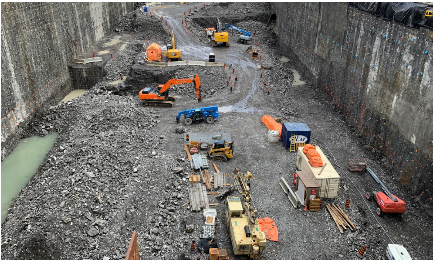
Excavation Work at Parliamentary Precinct
