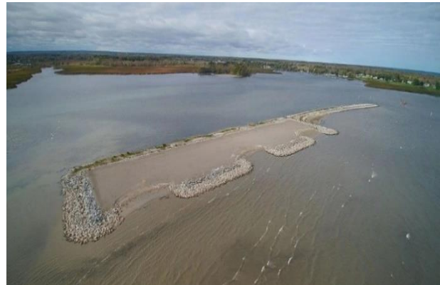
Figure 22. Braddock Bay barrier restoration.
