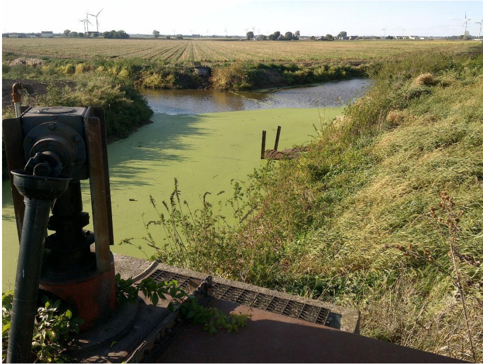
Figure 110: In Rondeau Bay (10RBY), dyke and pump system regulates water level near agricultural lands.
